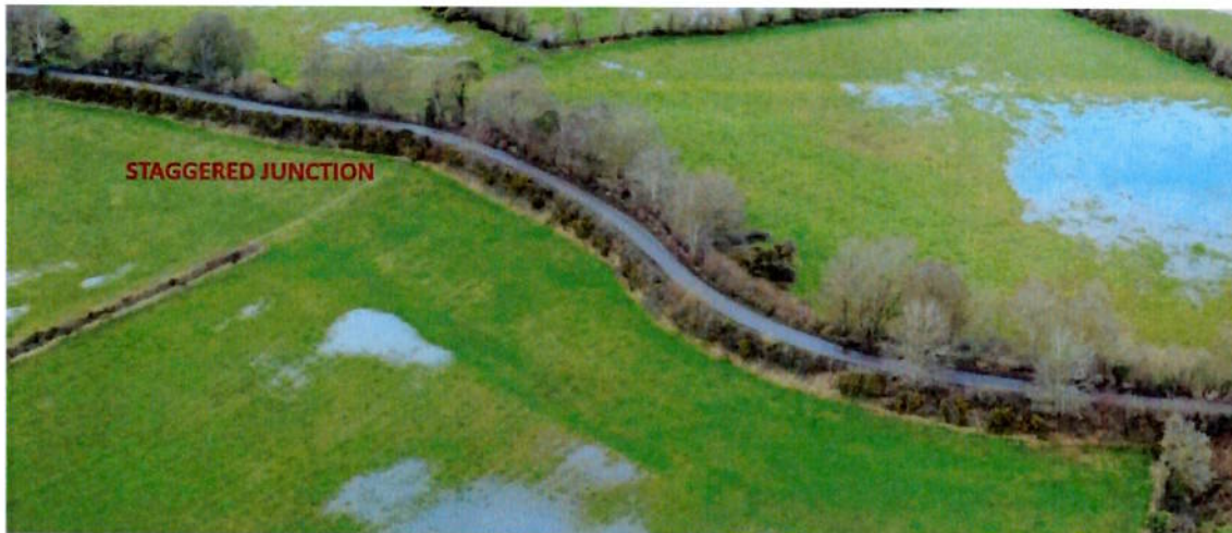
View of the proposed staggered junction over the elevated L8763 esker ridge.
